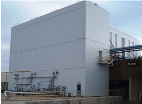
Multi-Purpose Plant Building
