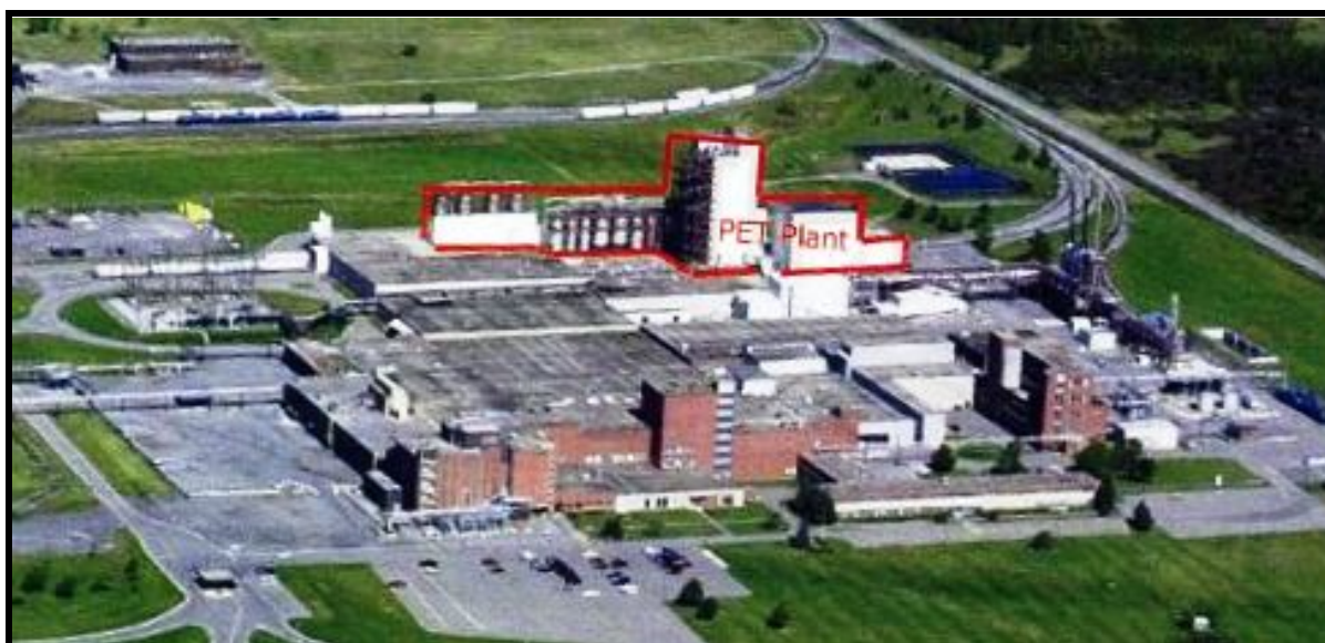
Aerial View of Entire Facility
