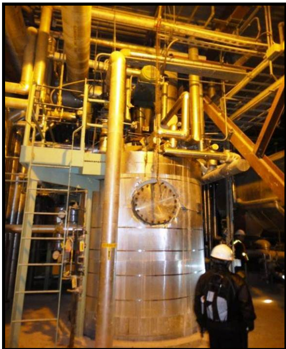
CP4 Primary Esterifier
