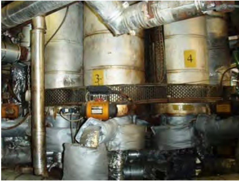
Distillation Column Steam Candles
