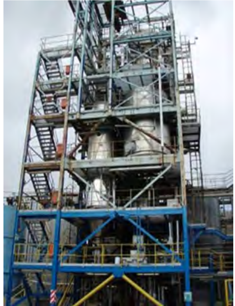
Luwa Evaporator Structure
